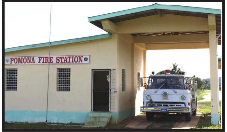
One of the new fire-stations, this one in Pomona, Stann Creek
