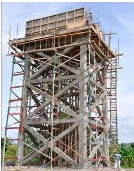
New Santa Familia Village 20,000 gallon tank under construction
