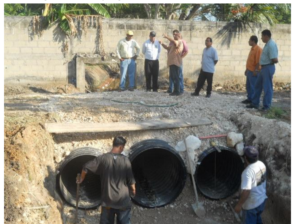
The New Outlet Across 1st Street - A 3 feet 6 inch culvert in the middle and two smaller 3 feet on both sides
