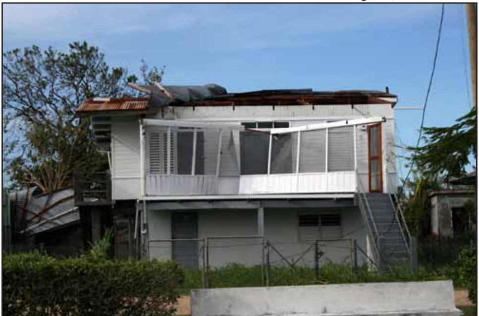
Lots of work ahead to restore this home to its former state, as it lost a good portion of its roof and sustained damage to its front verandah.
