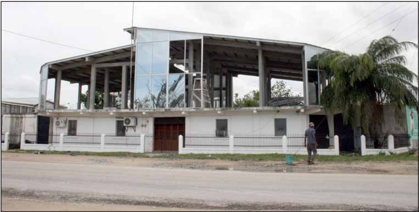
Total blowout in Corozal at the famous “crystal palace” (residence of former Social Security Board head Narda Garcia) as flying debris shattered all the plate glass windows during the hurricane, leaving only its skeletal frame.
