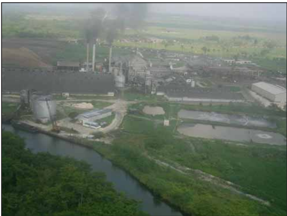
The BSI sugar factory at Tower Hill reduces the biological oxygen demand (BOD) of its effluent in treatment ponds before releasing it to the new river, but also causes thermal pollution from its condenser cooling water.
