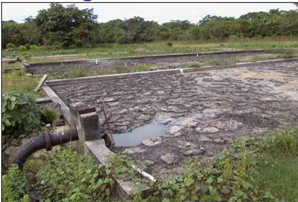
Mucked up mess! Non-functional Belmopan treatment plant forces raw sewage directly into the Belize River.
