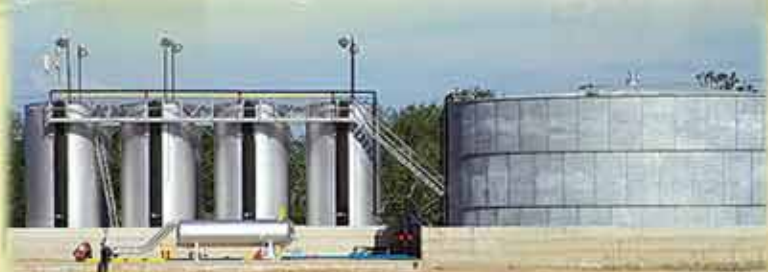
Separation unit and storage tanks at Iguana Creek
