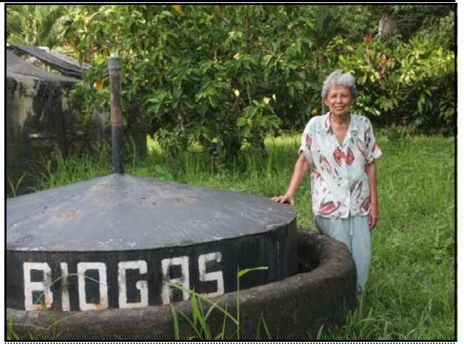
Yvonne shows the biogas collection chamber
