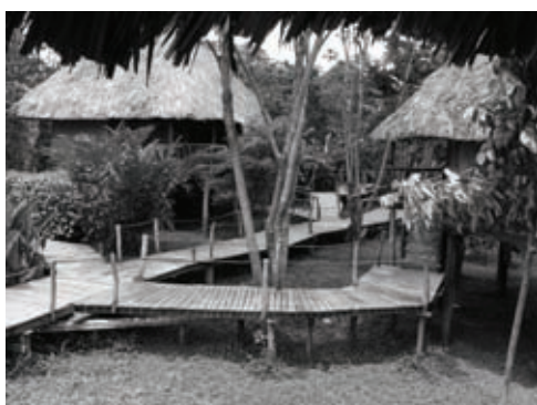
Raised walkways at Cotton Tree Lodge
