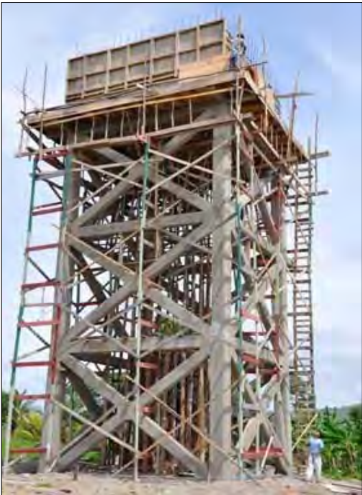
New Santa Familia Village 20,000 gallon tank under construction.
