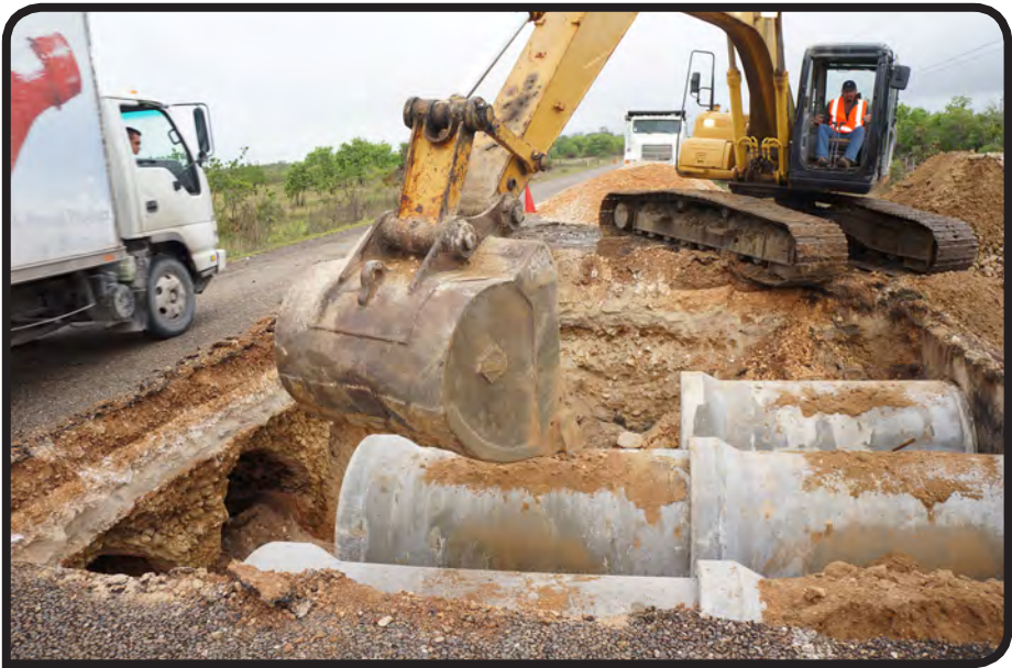
Portion of Road being excavated for installment of new culverts
