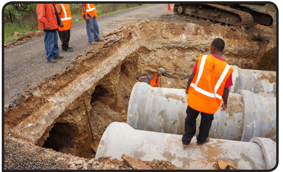
The new culverts being installed on Burrell Boom - Hattieville Road
