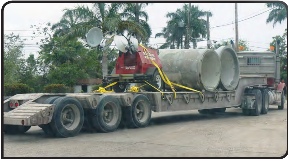
The new cement culverts being transported to the site
