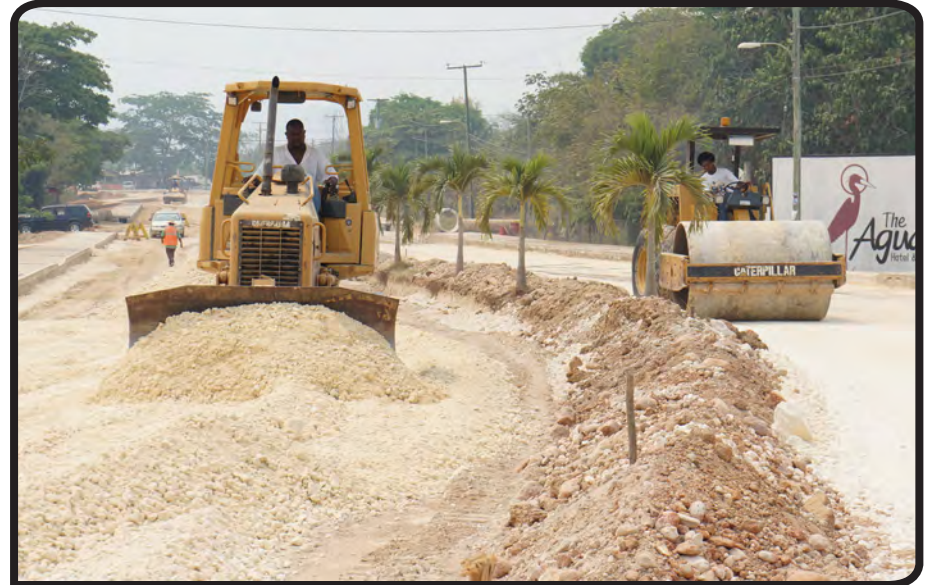
Bulldozer and Roller preparing re-shaping Loma Luz Boulevard
