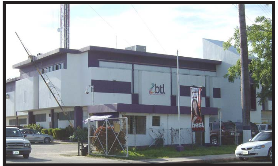
Belize Telemedia Corporate Headquarters
