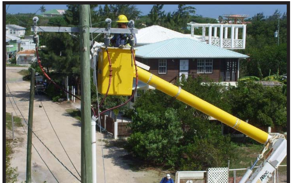
Belize Electricity Limited Technicians at Work
